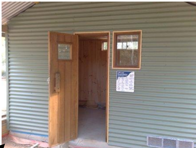
Another view of the nearly completed sauna.
